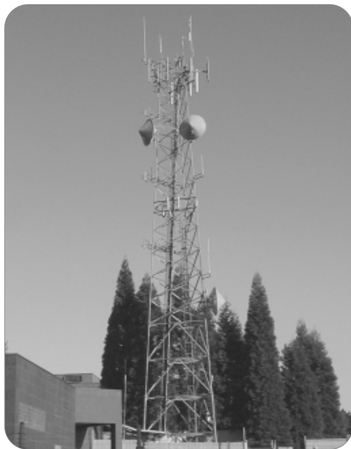
► Figure 1: Sign of the times: Here is a site with nearly thirty separate communications antennas mounted on the same tower as the cellular and PCS systems. With this many signals present in a small space, there is a much greater chance of them interfering with one another.
